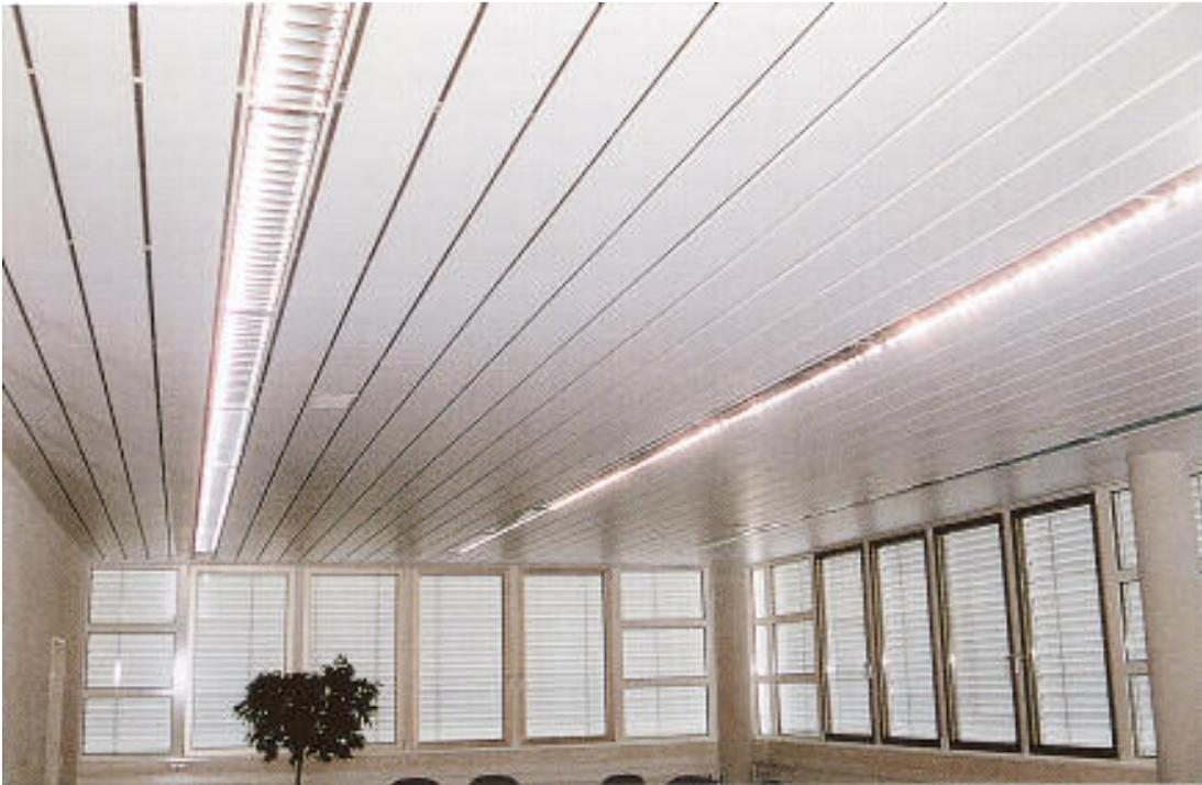
OFFICE BUILDING, ULM, GERMANY
